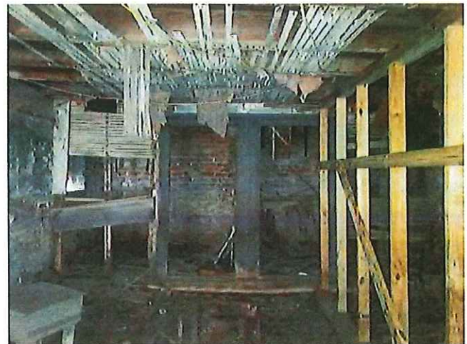
Cellar with shoring at right.
