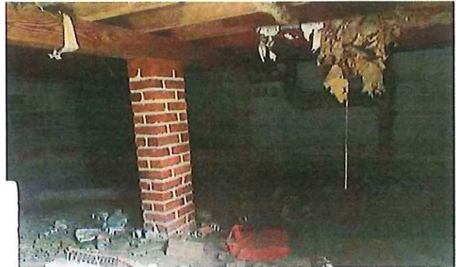
Crawlspace under 1940s addition.
