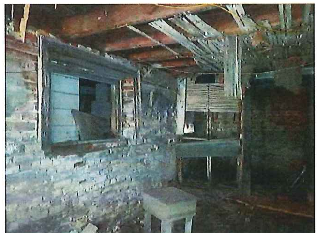
The cellar has remnants of finishes for restoration.
